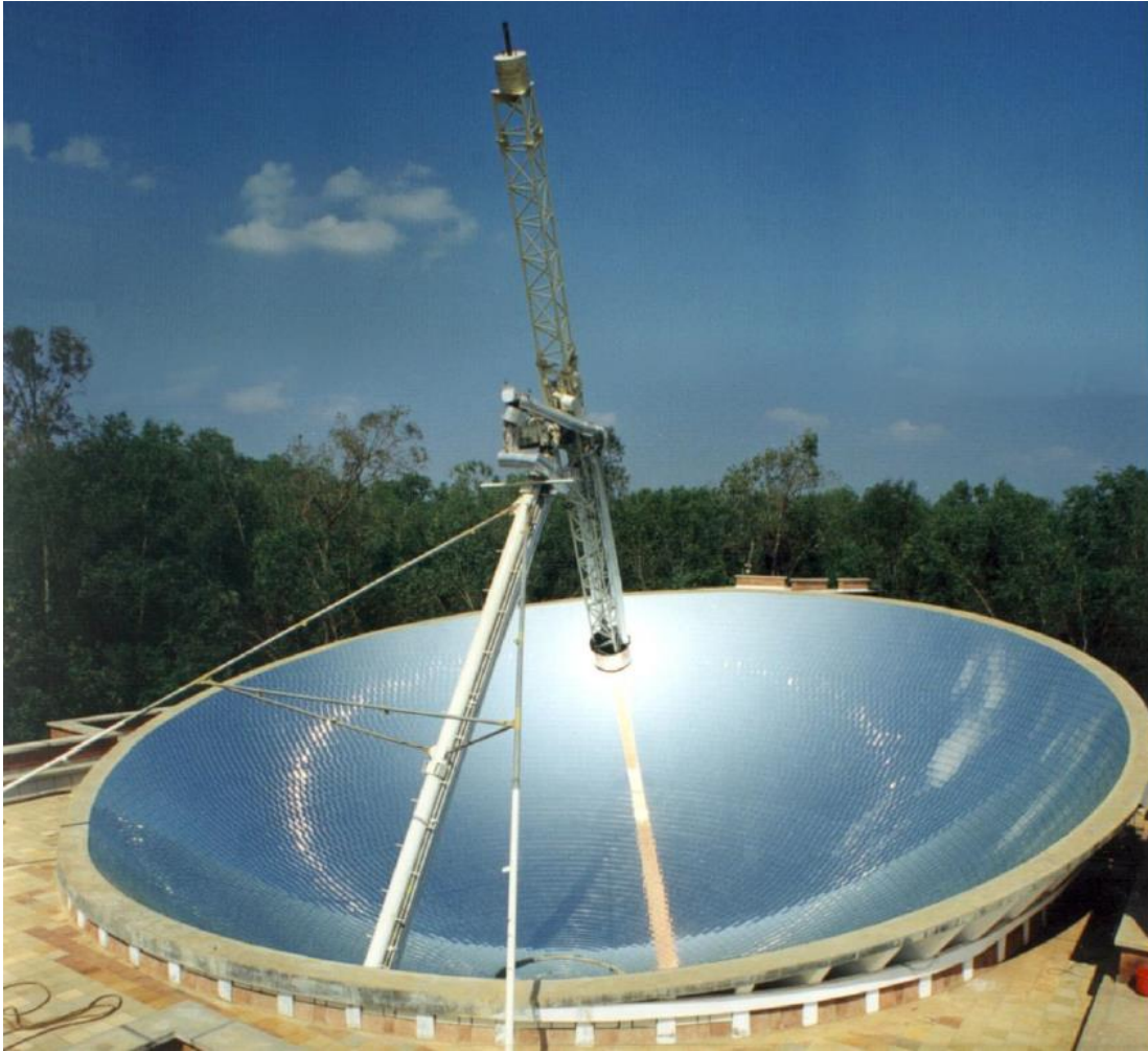
Figure 19: Solar bowl at Auroville/India during operation [29].
